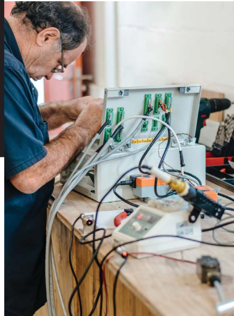
Dirk Streicher at work in the laboratory
